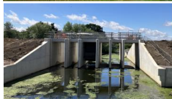
Images of scheme progress from the River Roding Project website
